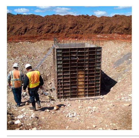
The Roaring Forks club lift station at Basalt Colorado was designed to include Xypex Bio-San C500 in the concrete mix. This provides both protection against microbial induced corrosion and watertight, chemically protected concrete.
